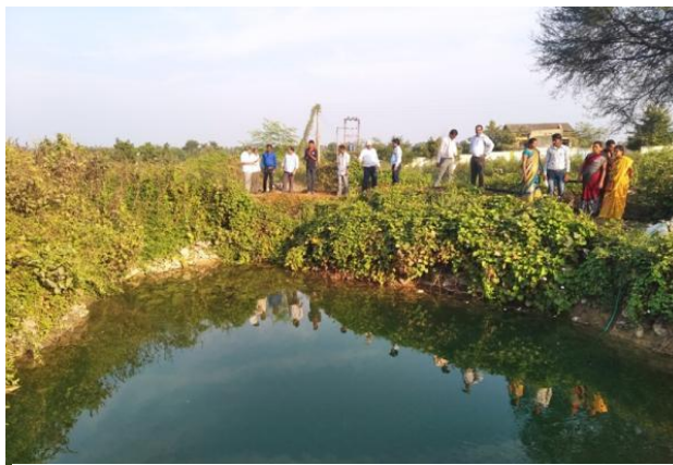
The rainwater harvesting structure in the village Nimbarda during the month of November 2019
