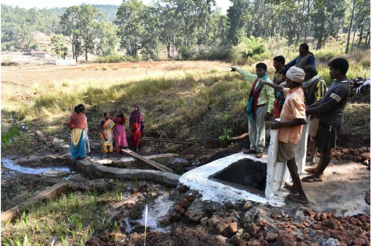
In two filter chambers, net has been fixed. Above this net, there is one layer of big sized boulders, one layer of small round shaped boulders and finally at the top, there is a layer of sand.
